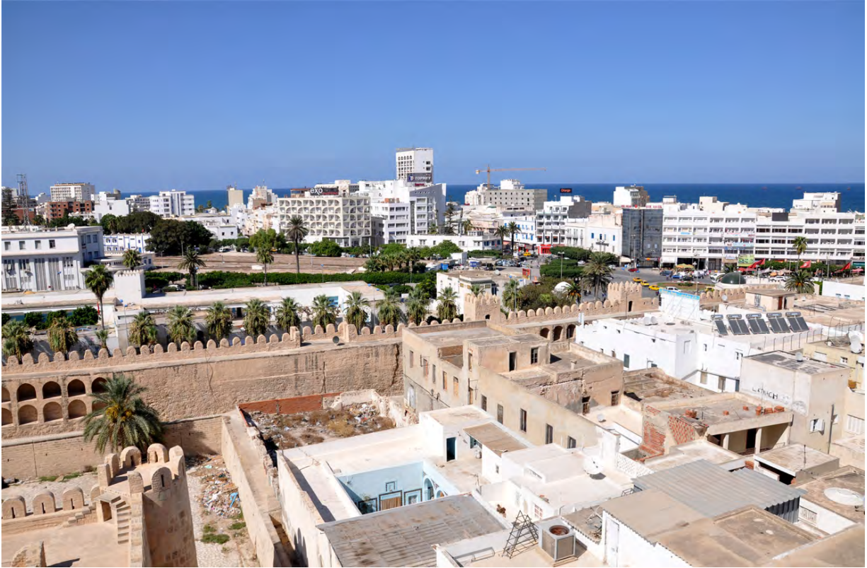
Figure 16.2 The increasing urbanization of Sousse.
